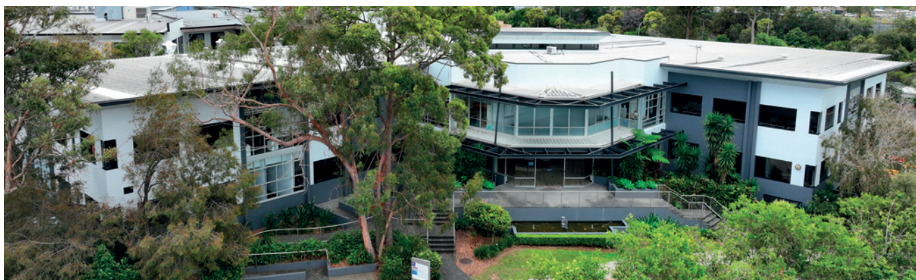
The new custom-built toxicology facility in Brisbane
